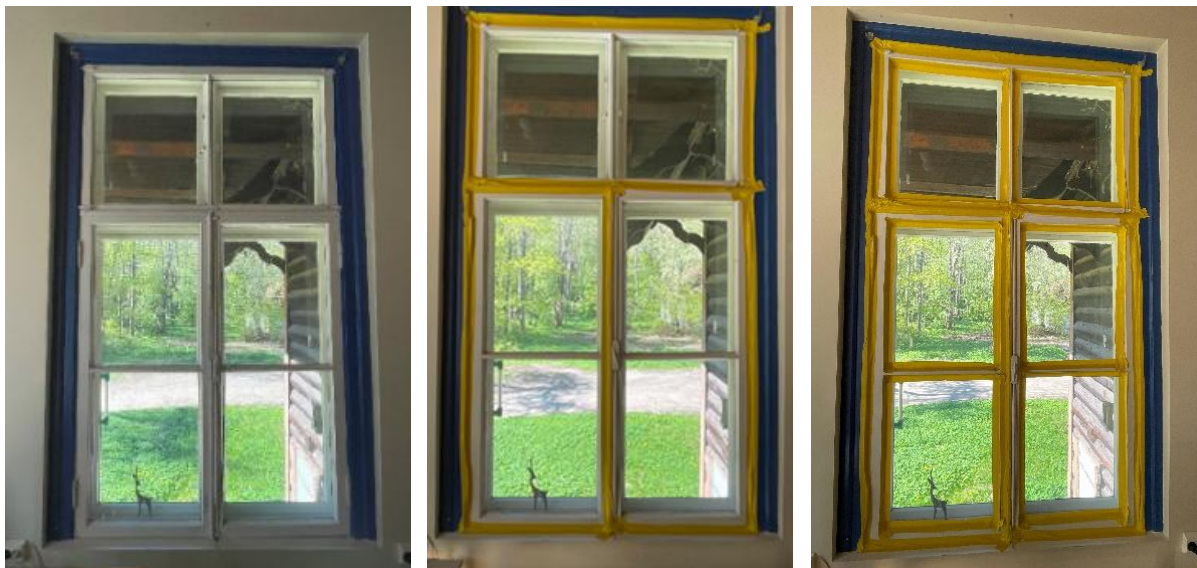
Figure 39 Air permeability at 50 Pa. Original (left) – 32,94 m³/(h·m²). Taped frame-jamb joint (middle) – 1,91 m³/(h·m²). Taped frame-jamb and frame-glass joints – 1,27 m³/(h·m²)
