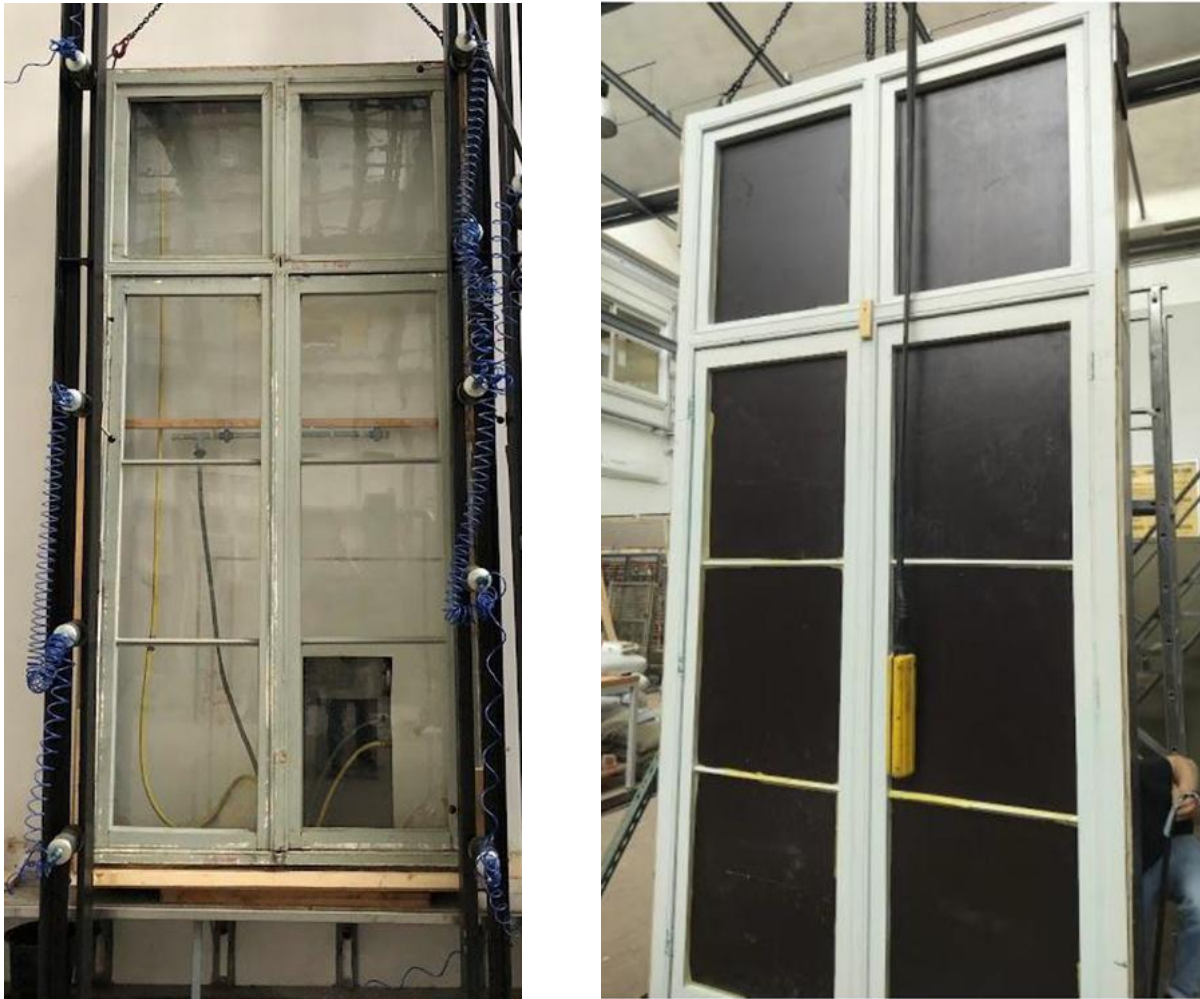
Figure 5 Original and refurbished window Rozier
