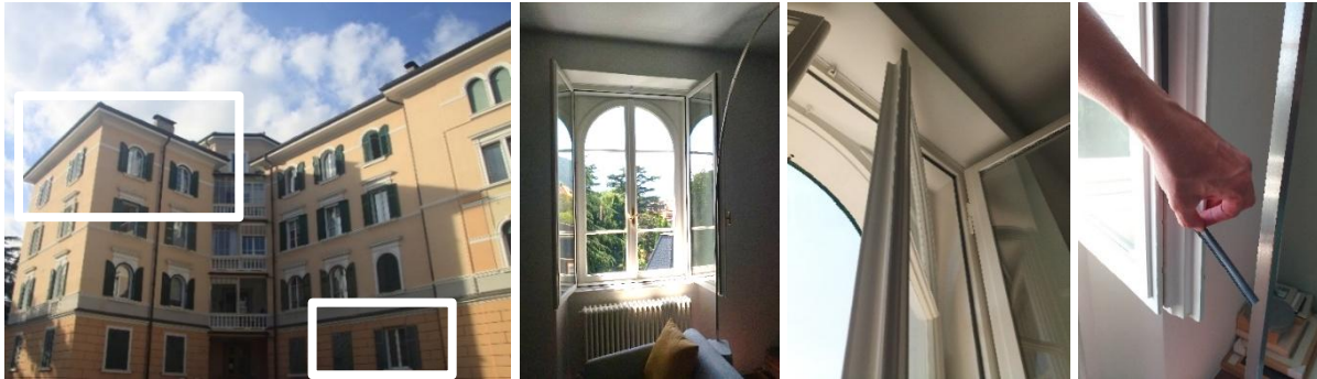
Figure 48 Railway Workers House in Bolzano/IT, with indication of the measured windows. Photos of the refurbished window with “Wolfsrachen” and the sealing of the inner window.
