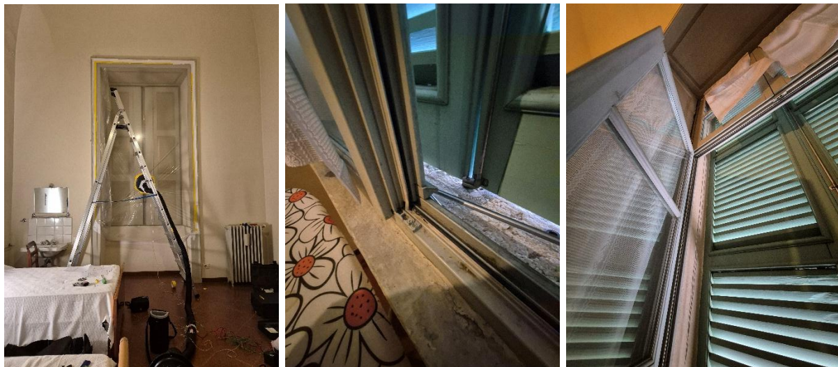
Figure 46 Air-tightness measurement build up at Palazzo Vescovile and detail of window showing double glazing and exterior shutters
